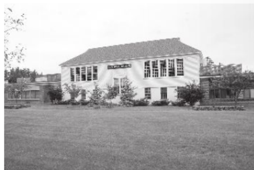
Town Hall, as seen today, now envelops the original school, while the rooms to the elementary school can be seen to the right. Town Hall entrance is to the left, and the Police Station is behind Town Hall
