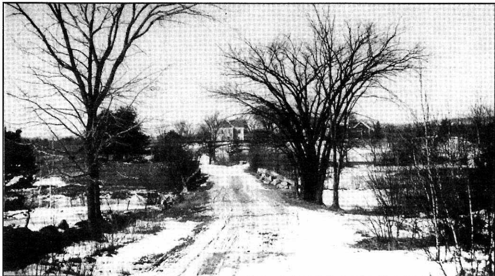
Center Bridge about 1900. In the background is Pilgrim Hall.
