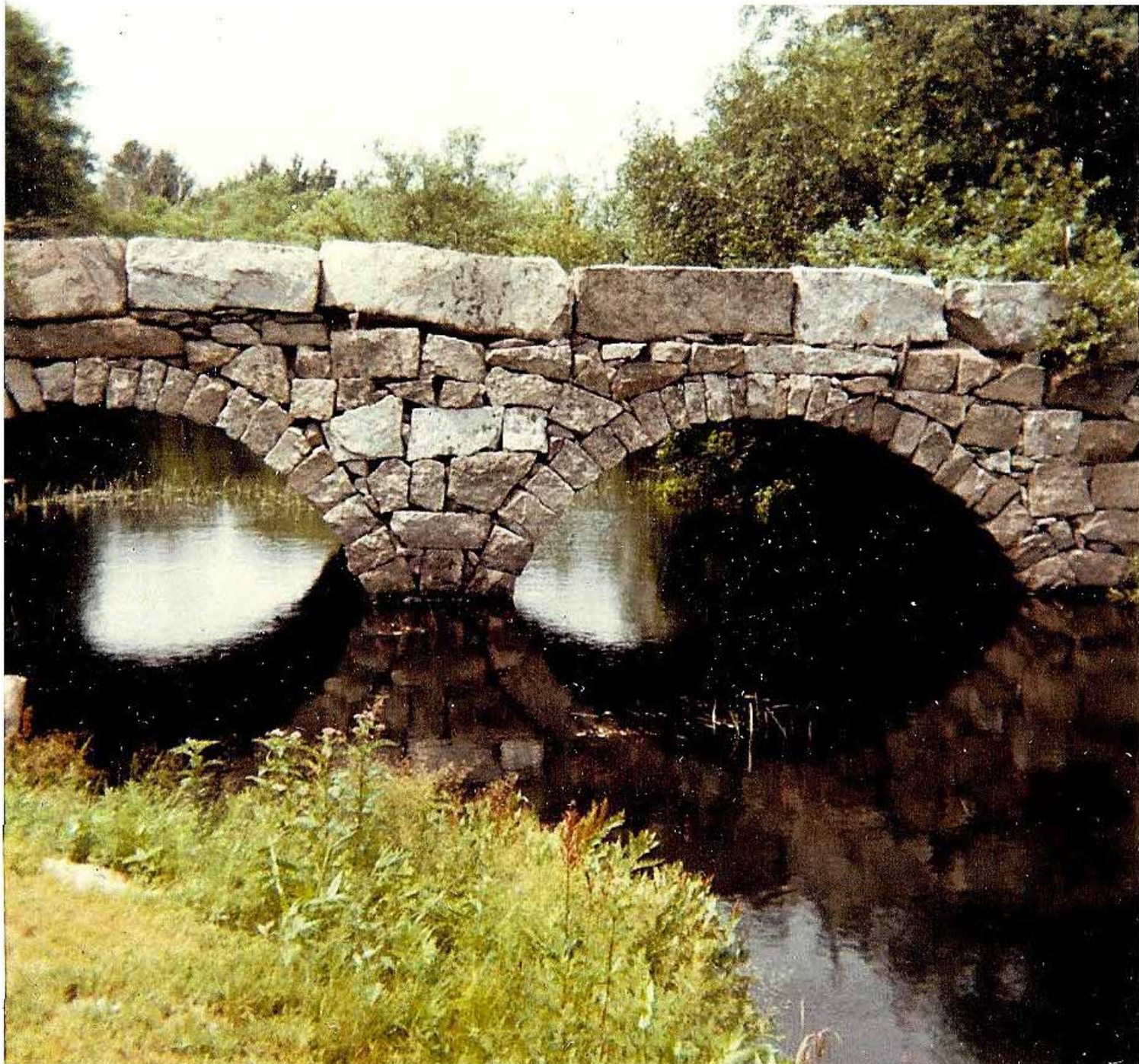
Abbot Bridge: The oldest mortar free double arch bridge in New Hampshire.
