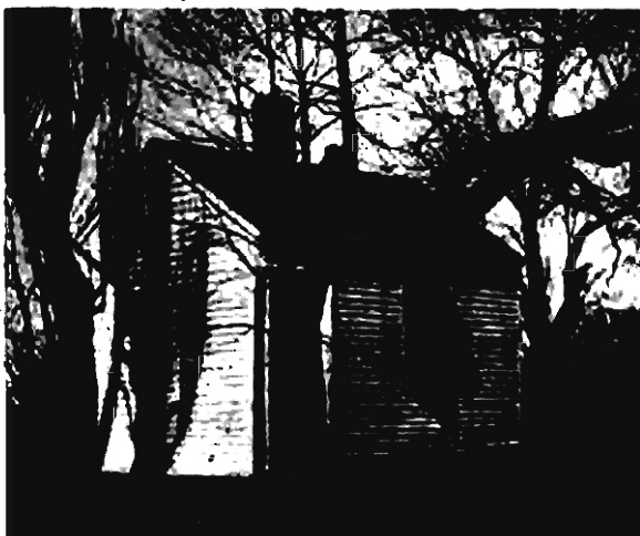
Toll House of Old Middlesex Canal, Middlesex Village.
